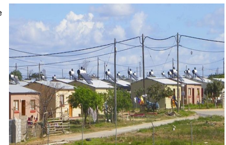
Figure 6: South Africa’s first mass greening project—the equipping of 70,000 low income households with solar water heater systems
