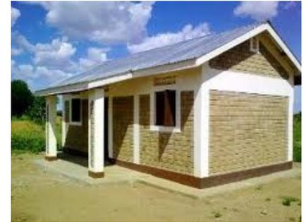
Figure 1: Building Constructed using Interlocking Blocks
